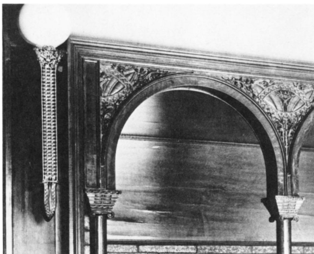
Fig. 1. Detail, vestibule, Winslow House, River Forest, Ill., 1894, Wright (photo: Chicago Architectural Photograph Co.).
